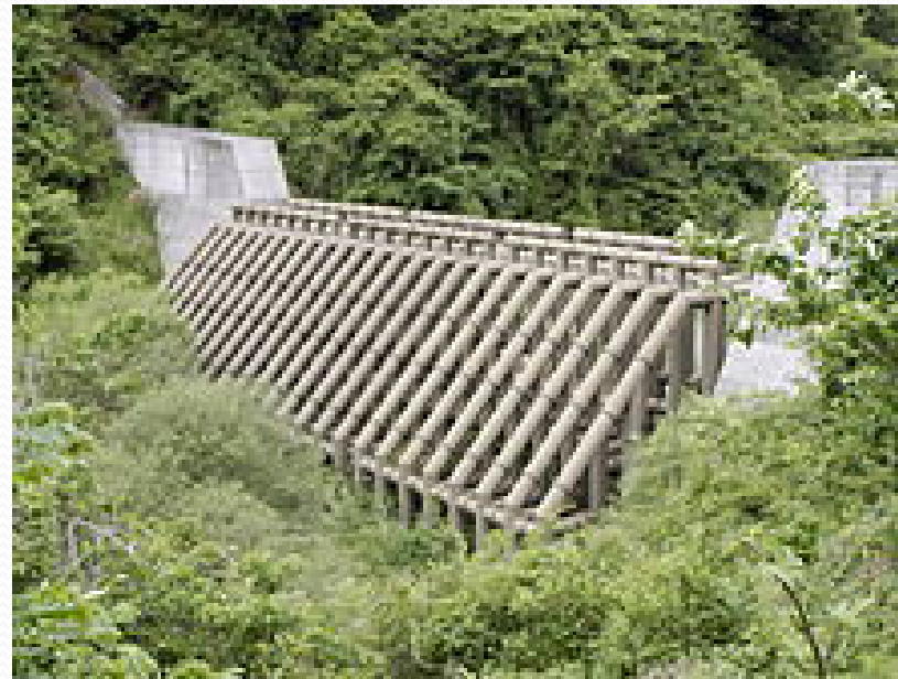
A steel check dam
